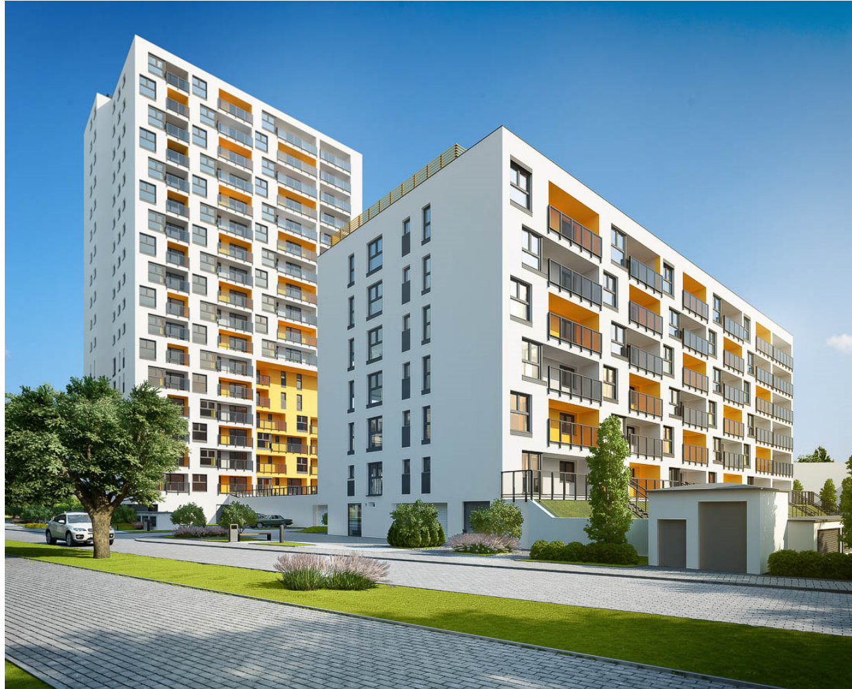
Apartamenty Innova, Wrocław (Poland). Breaking ground: November 2014.
